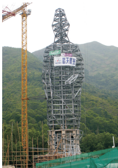
The completed steel frame of Guan Yin statue at Tsz Shan Monastery
