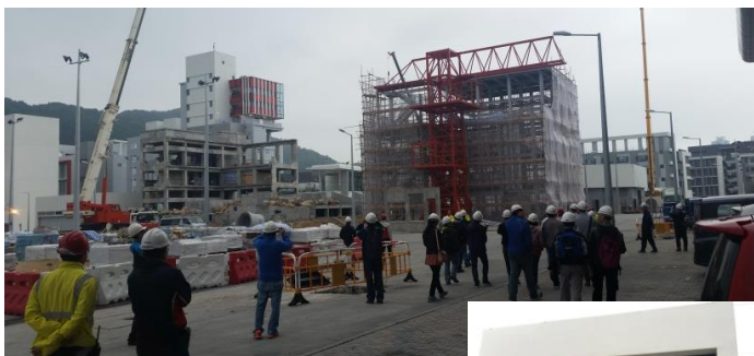
Buildings and tunnel facility
