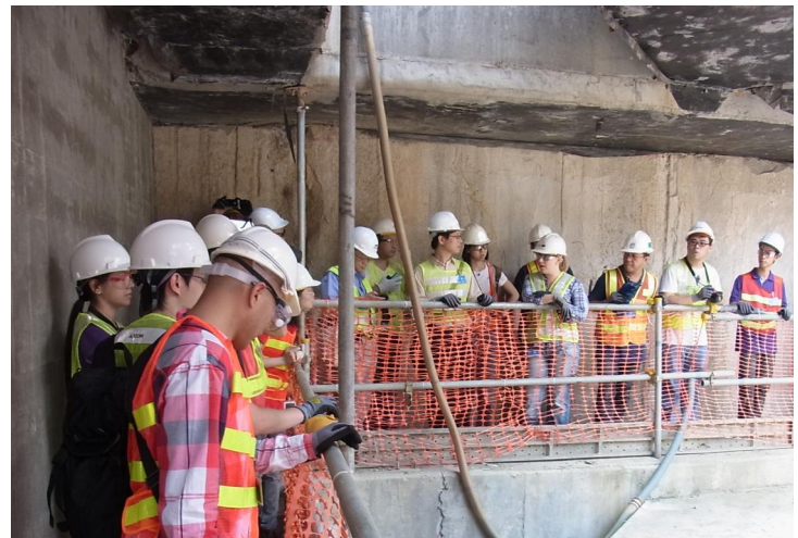
The site of West Kowloon Terminus Approach Tunnels (North)
