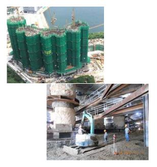
In this site visit, the participants will see the ELS works, semi-top down basement construction and associated connection details at bored piles and socketed H-piles.
